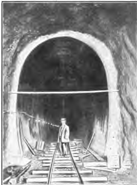
New York City is spending $350,000,000 to have a pure and abundant water supply. This is the tunnel which will bring the water from the Catskill Mountains to New York City.
